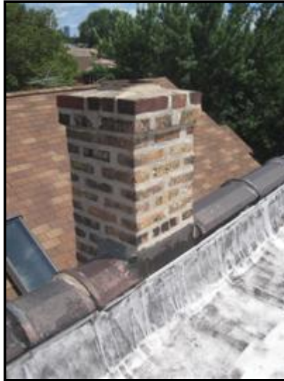
A. Picture 1 North chimney - does not appear active
