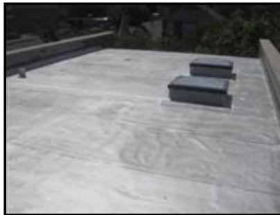
E. Picture 3 General view of roof
